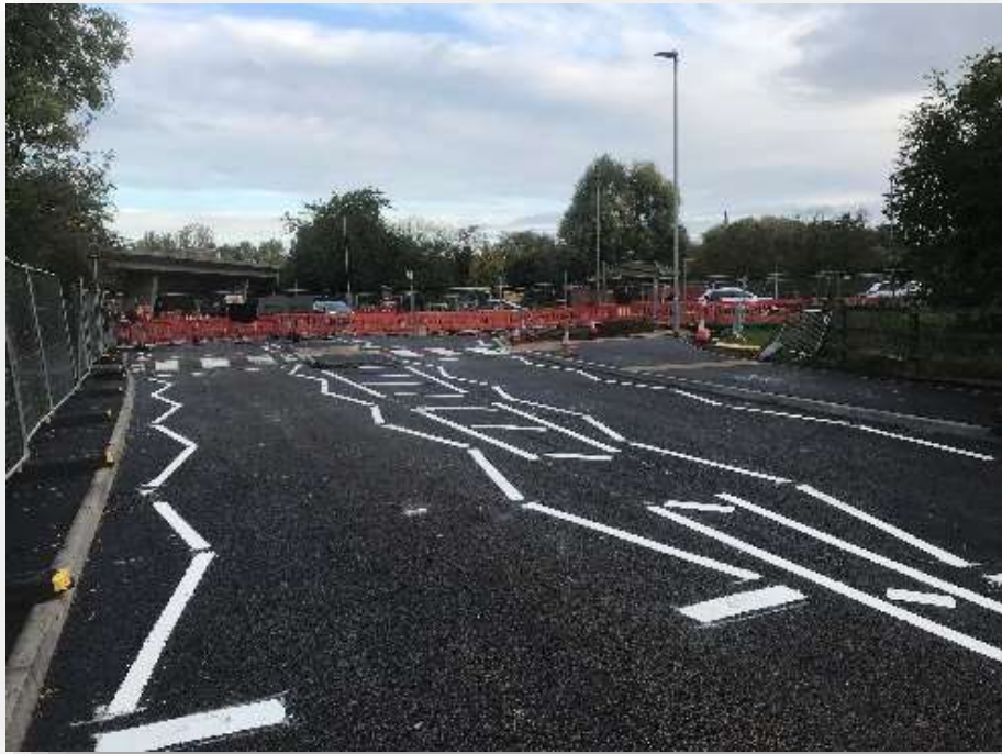
Whittlesey Road Pedestrian Crossing
