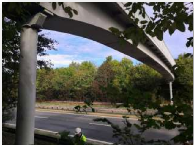
APV Baker Footbridge
