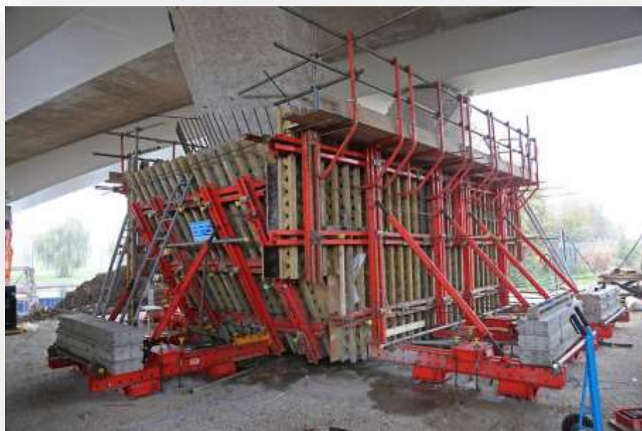
Construction of the Concrete Jacket on Nene Bridge Piers
